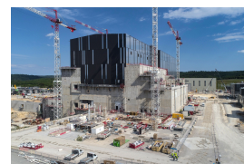
Figure 2. The Tokamak Complex at the ITER Site (from iter.org )
